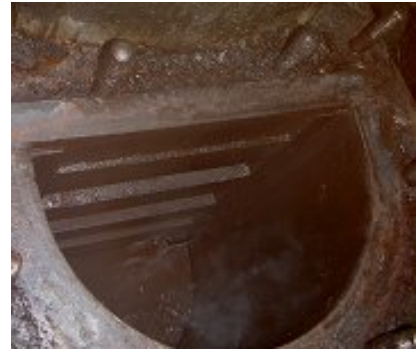
Inside of valve chest showing port face
