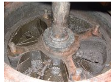
Top plate of piston removed showing jumble of metal and contamination (7,8)
