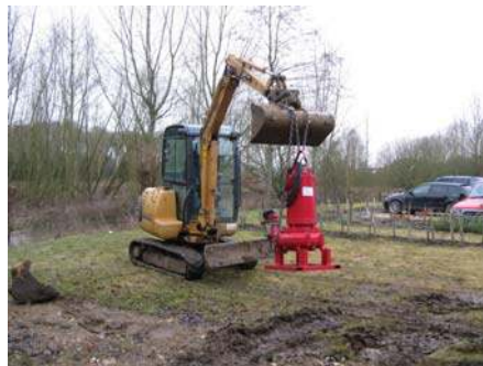
Submersible is lifted into position in a recess in the river bank
