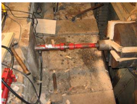
Pressing the gudgeon and new wedges into place
