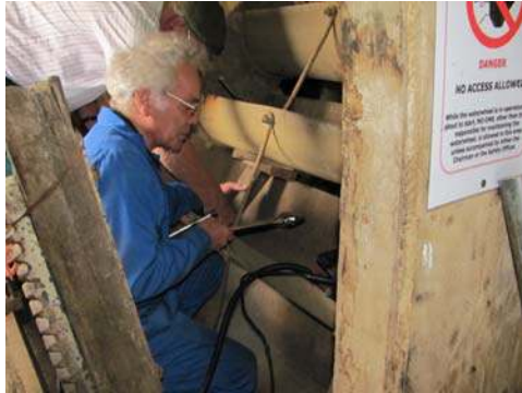
Ron Winfield welds a metal plate to repair one of three buckets
