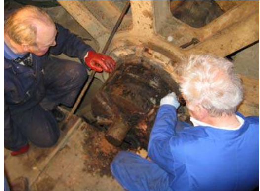
Henry Sparrowhawk and Ron Winfield examine the gudgeon retaining wedges
