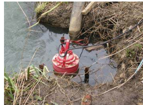
Submersible is lifted into position in a recess in the river bank
