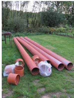
10" pipe awaits laying but was later exchanged for a smaller diameter
