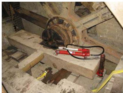
Jacking the axle into alignment
