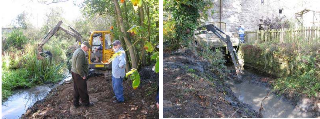
Excavating the tail race channel
