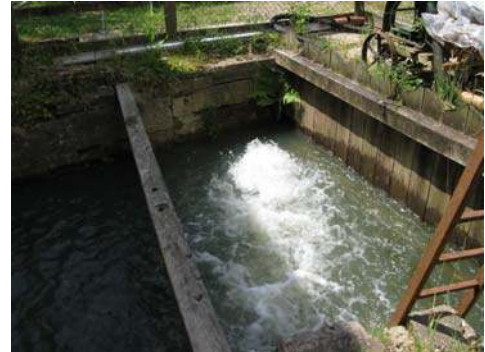
Water surges into the head pond from the new submersible
