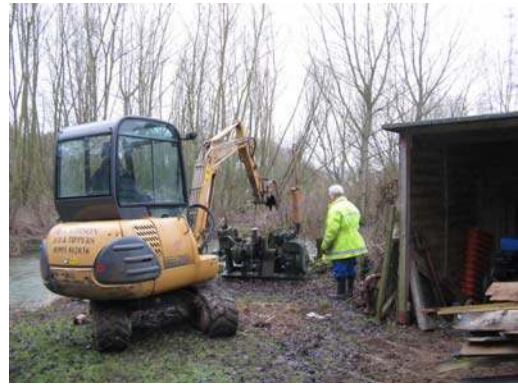
Digger driver lifts Joe Curryer's diesel pump out of the way
