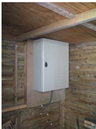
Three-phase electrical supply being paid to the end of the 'old' barn engine shed
