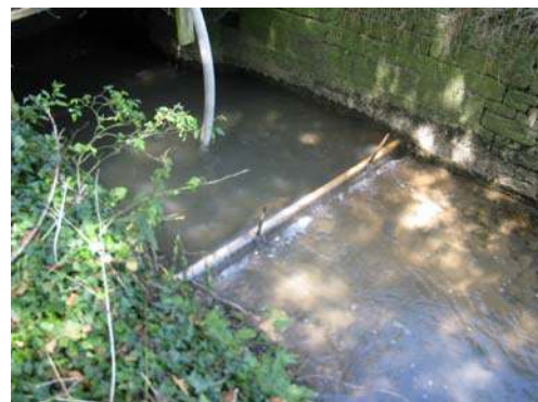
Board across tail race to retain water under the wheel
