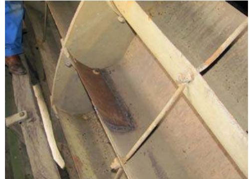
Ron Winfield welds a metal plate to repair one of three buckets
