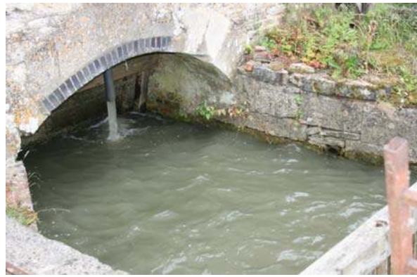
A good level in the head race needed to turn the wheel – we found that it was more flow that was really required
