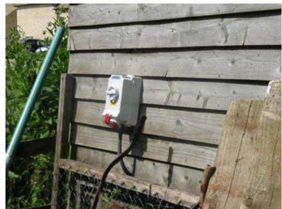
Three-phase electrical supply being paid to the end of the 'old' barn engine shed
