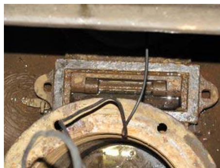
Cold well bottom flap valve seen from above
