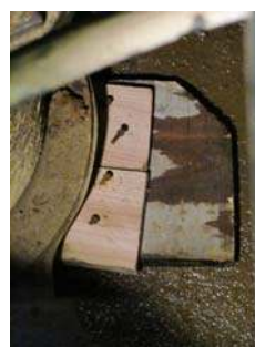
Wooden wedges under manifold
