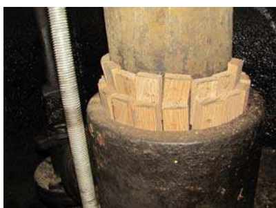
New oak wedges for condenser seal
