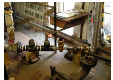
New steam main from traction engine to beam engine
