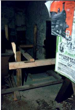
Frame locating holding down bolts
