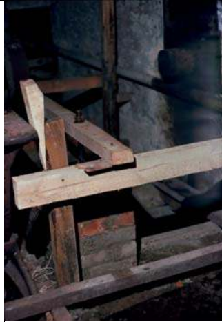
Plinth partly built
