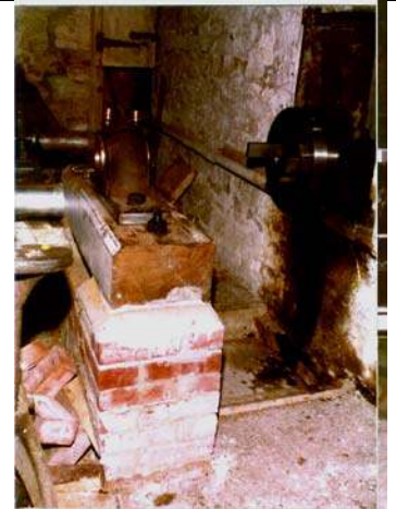
Plinth with bearing located and wedges in couplina beina fitted
