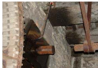
End of line shaft and support for disengaged gear wheel
