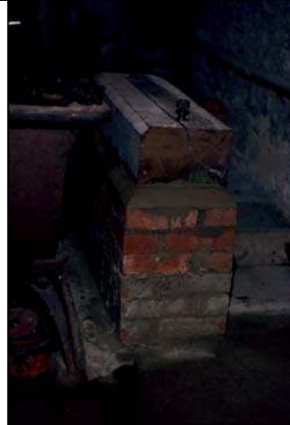
Completed plinth with the oak beam above
