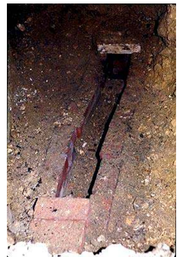
Brick lined drain under plinth carrying new bearing
