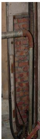
Slot in engine room wall
